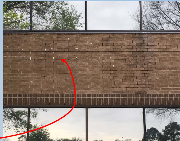
Gap between window and frame
