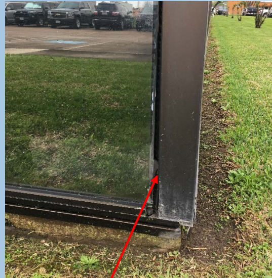
Gap between window and frame
