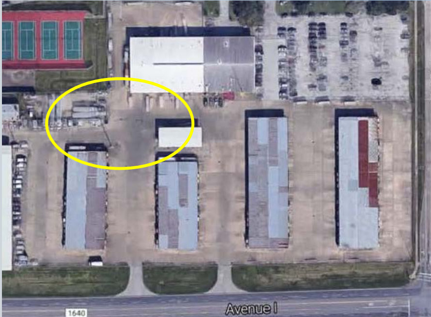
Lamar Campus Transportation Fueling and Tanks to match Fulshear
