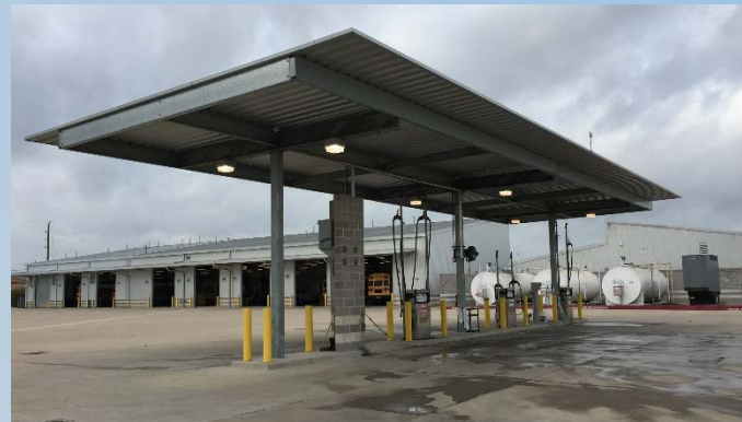
Fulshear Transportation Facility
