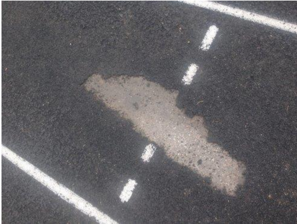
Source: Review Team's Athletic Facilities Inspections, April 2017.
