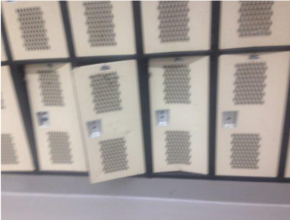
Source: Review Team's Athletic Facilities Inspections, April 2017.
