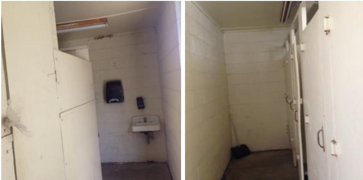
Source: Review Team's Athletic Facilities Inspections, April 2017.
