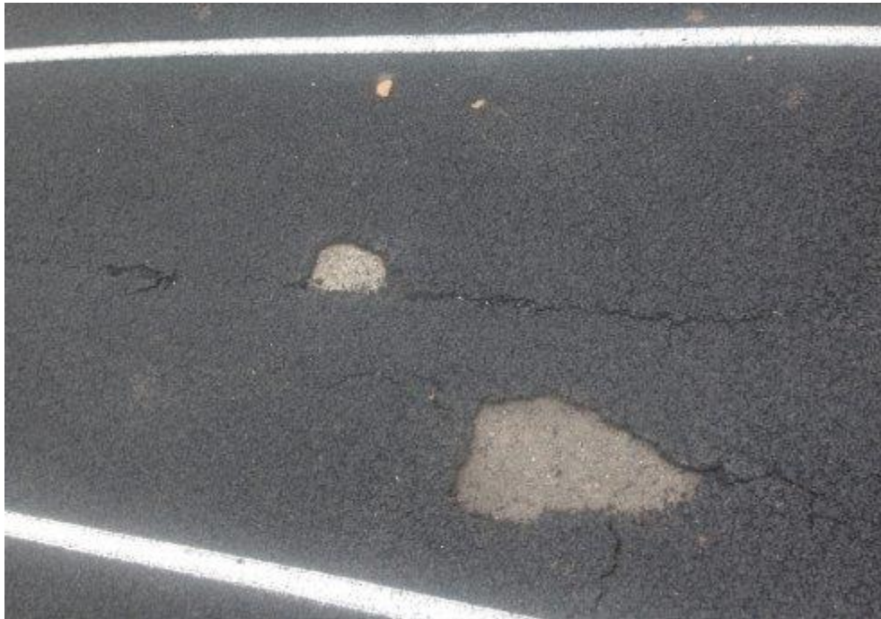
Source: Review Team's Athletic Facilities Inspections, April 2017.
